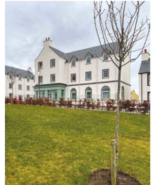
Left: Plan of Cairnhill Centre, above: The Lounge is moving to Quarryline Street
